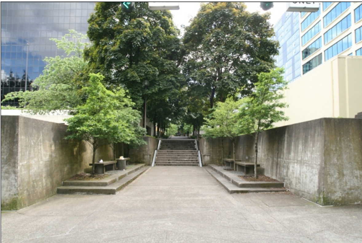
Photo 12 of 14: Third Avenue Pedestrian Mall from Market Street, camera facing south
