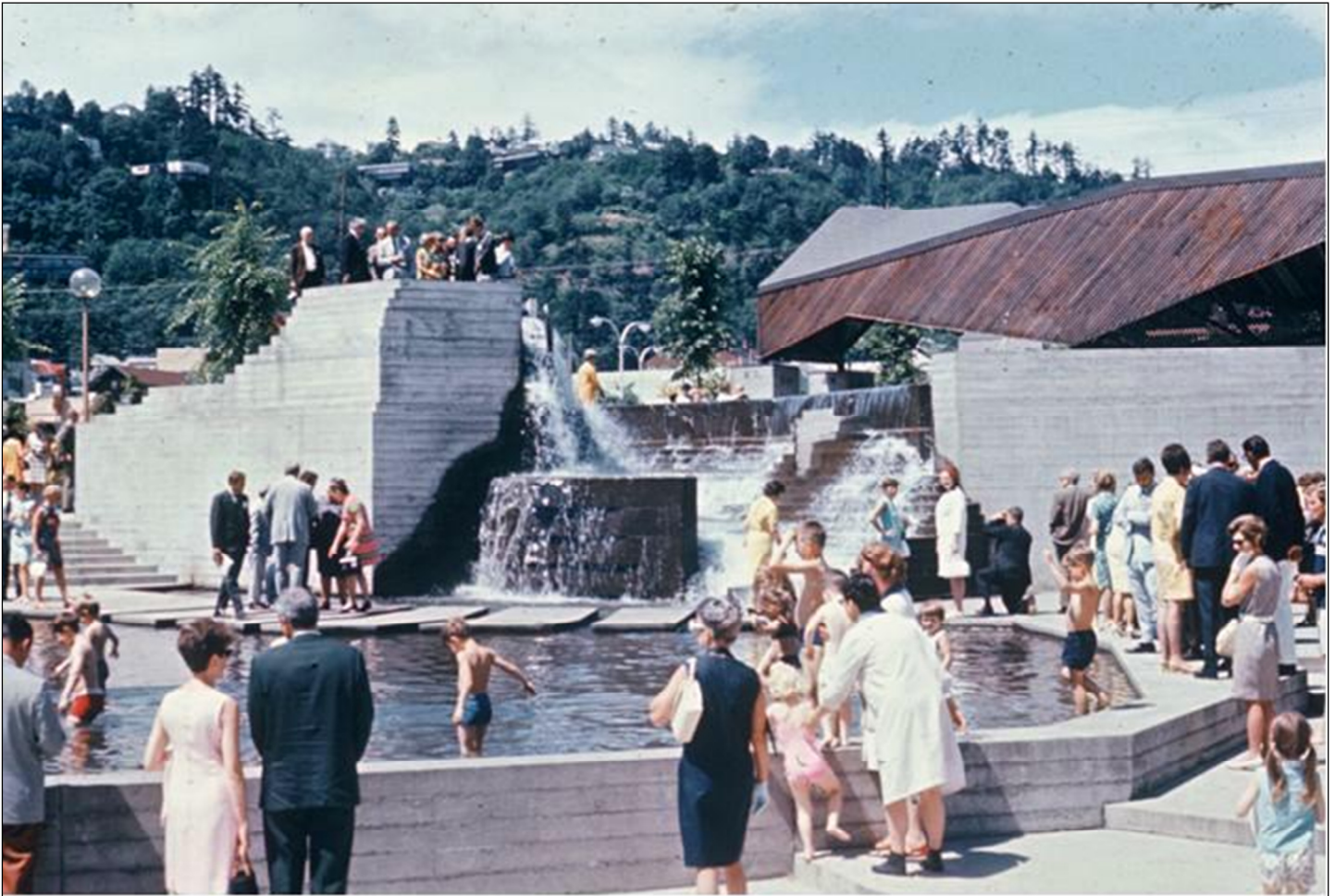
Figure 11: Lovejoy Fountain Park, 1966 (Courtesy of the Portland Development Commission)
