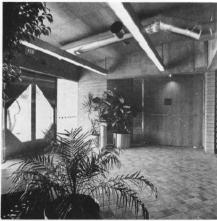
Mesquite Branch, Phoenix Public Library, Phoenix, Arizona, 1979–82. This 10,000 square foot public library uses a simple 45 degree geometry in massing and plan. The main reading room has a very human scale defined by a ceiling of large exposed precast concrete beams, natural re-sawn fir plywood sheeting and sculptural galvanized metal ducts. Furnishings, graphics, and artwork selected by the architect give it a sense of design completeness.
